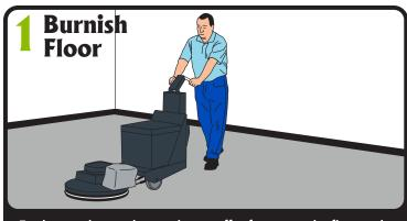
For better gloss and immediate traffic, force cure the floor with an 8,000-grit diamond pad followed by a white polishing pad to remove haze marks and produce a clear, crisp gloss.
