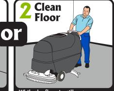
While the floor is still wet, use a 175 RPM swing machine or auto scrubber to clean the floor with a maroon surface prep pad.
