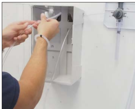
Connect the Rite-Connect pick-up tube assemblies.
