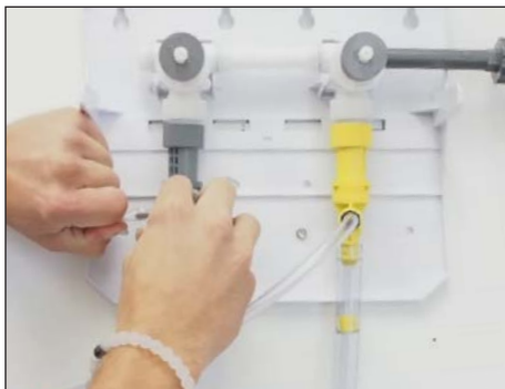
Remove pick-up tube assemblies.
