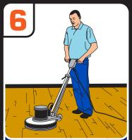
Lightly sand the floor with a Maroon SPP pad.
